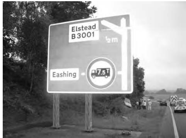
Figure 7. Accident with a Lattix signpost. The driver was unhurt and is standing near the car.
