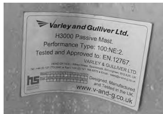
Figure 4. Varley and Gulliver Signpost Label on a passively safe signpost showing the EN12767 classification.
